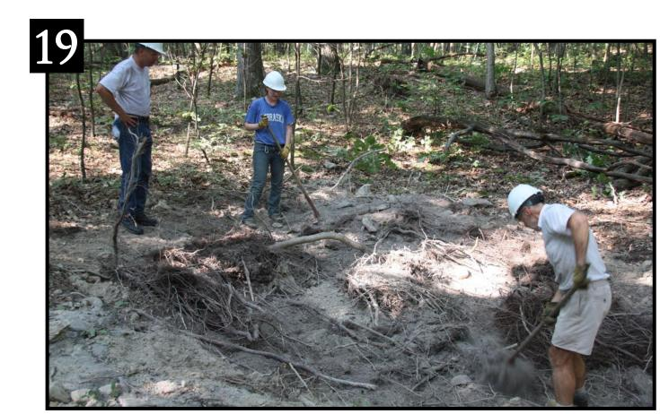
K. KING AND M. BERTRAM/ TNC The mineral soil (photo 9) was replaced and topped with 1 inch of topsoil (photo 7). Hand tools were used to smooth the upper edges of the basin.
