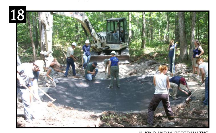
The second half of the liner was unrolled, secured, and covered with soil. Never allow
