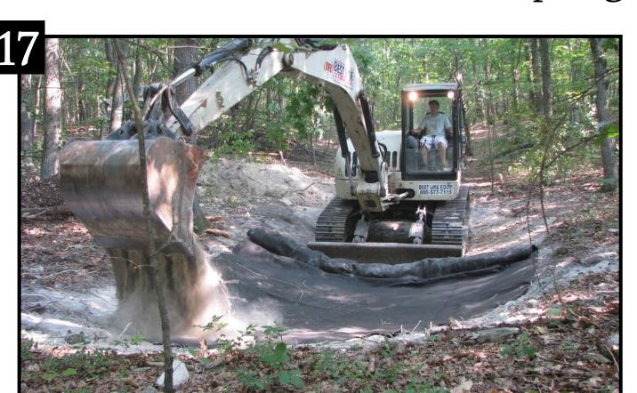
Rolling the liner allowed the excavator to drive closer to the secured half to replace soil.
