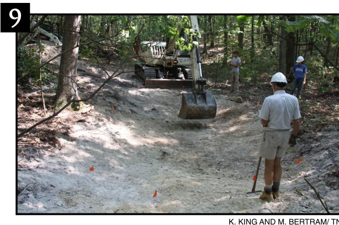
About 8 to 12 inches of mineral soil and rock were removed and set aside. A gradually sloped depression was shaped and compacted by the excavator.
