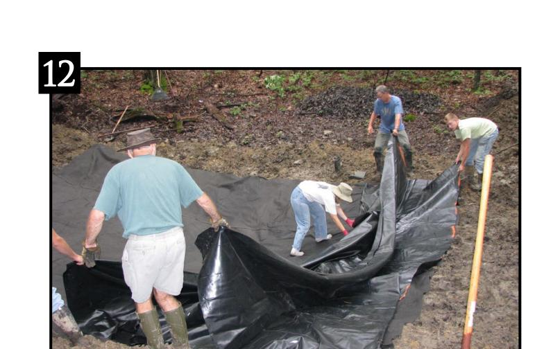
T. COLEMAN/ TNC The three liner layers were placed in the depression one at a time. The 30 mil aquatic-safe liner was protected on both sides by 16-ounce geo-textile pads.
