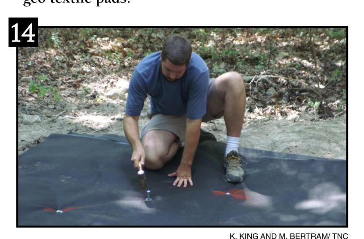
The three liner layers were held in place by 12inch galvanized steel spikes and washers. These were placed along the upper edge of the liner at the high water-mark indicated with spray paint.
