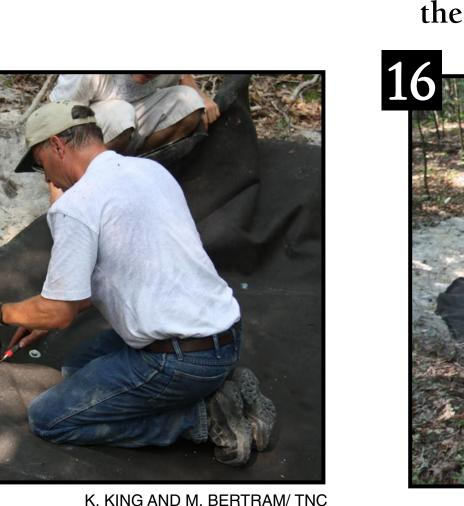
Once the liner was secured, excess material was trimmed from above the spikes.
