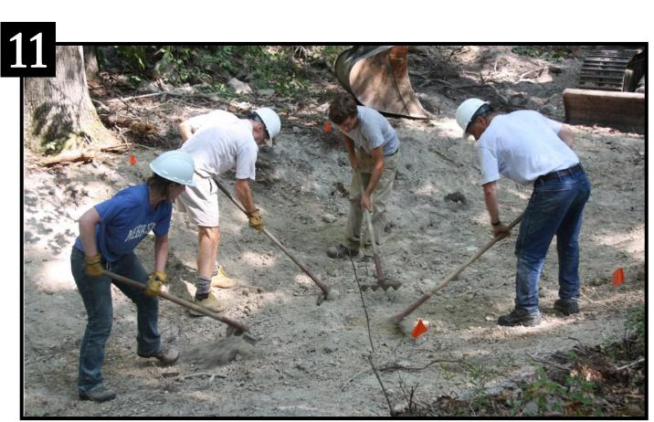
K. KING AND M. BERTRAM/ TNC The rough excavated depression was smoothed by raking sideways and uphill. It was important to remove any sharp rocks or sticks from the depression to prevent puncturing of the liner.
