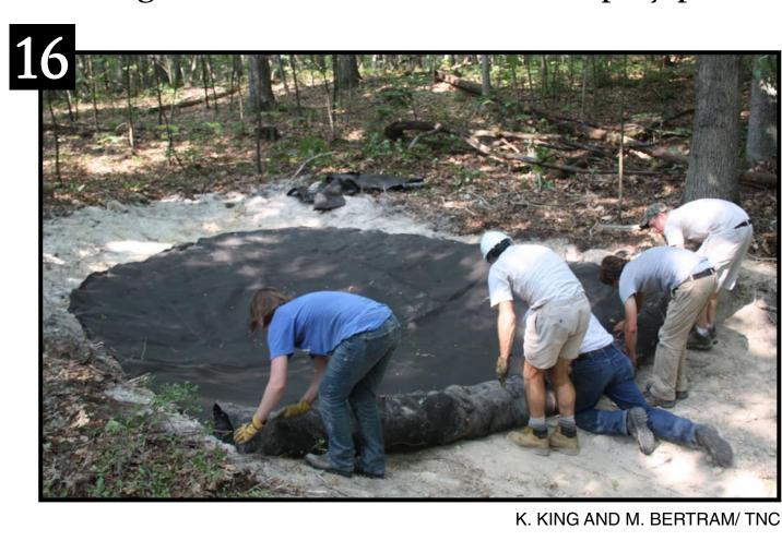
One half of the liner was secured, the other half rolled back.
