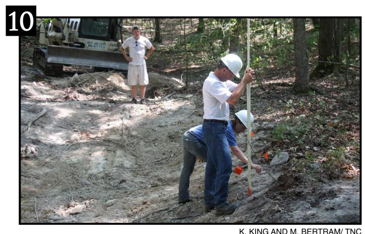
Target basin dimensions were marked and checked using the construction level and flagging.
