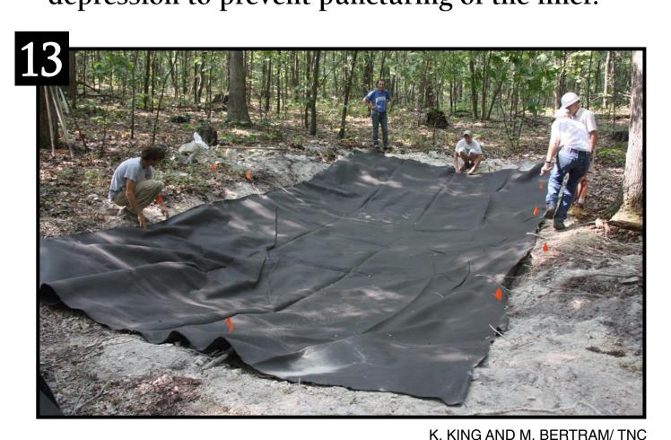
The orange flagging marked the high watermark of the pool and indicated placement of the liner and pads.
